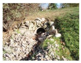
Debris in Mid-Berm Outlet-South Side
