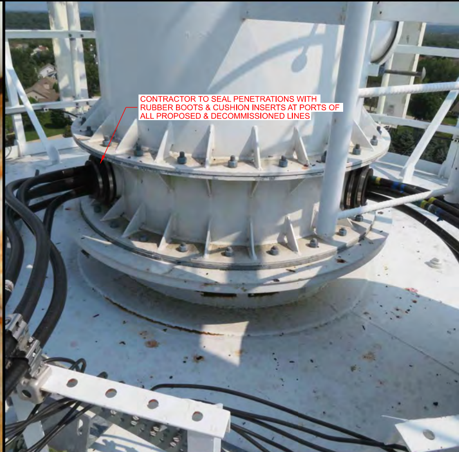
F CABLE PENETRATIONS AT TOWER ROOF
