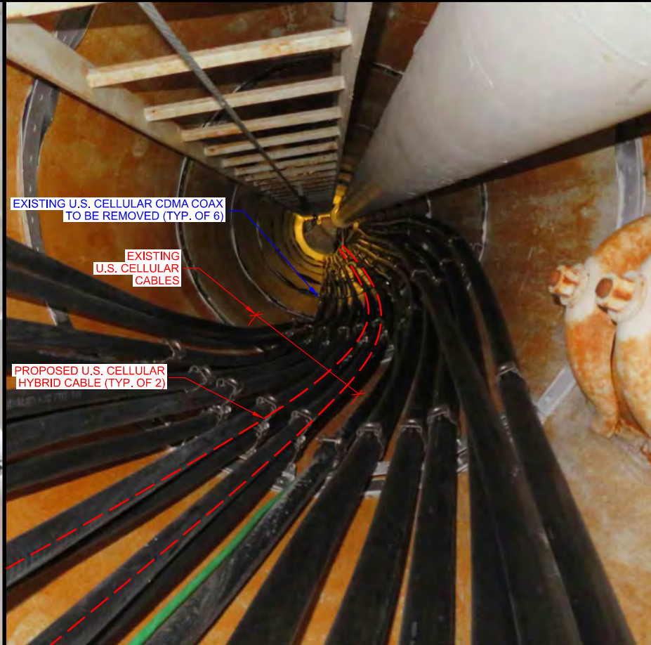
E CABLE ROUTE IN ACCESS TUBE
