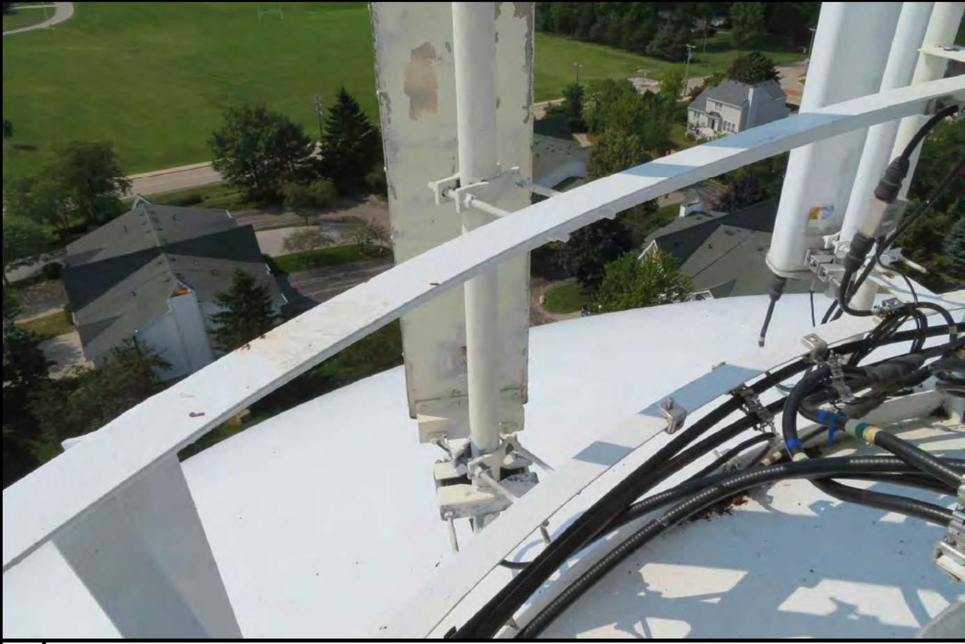
EXISTING ANTENNA MOUNTS
