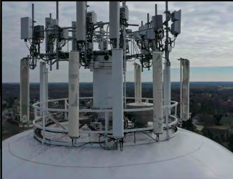
E U.S. CELLULAR GAMMA SECTOR ANTENNAS
