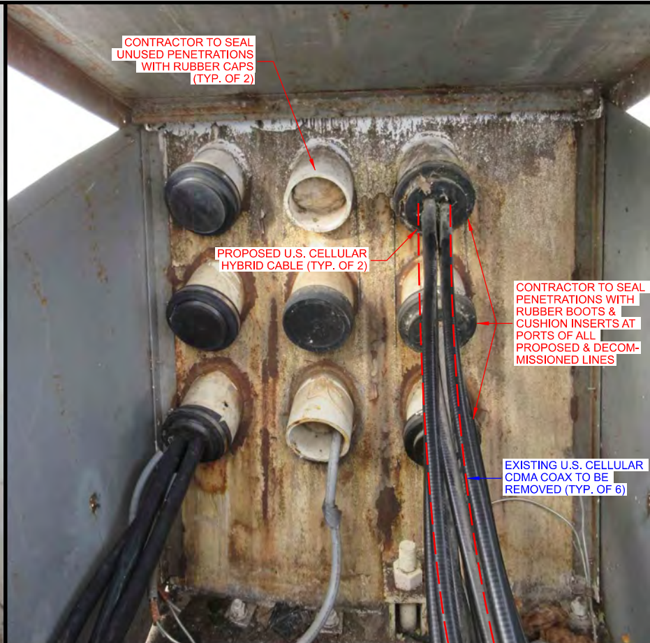
C LOWER TOWER PENETRATIONS
