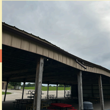
Support Posts Sinking (South Side) Impacting Gutter Function
