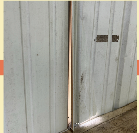
Siding has Punctures and Holes
