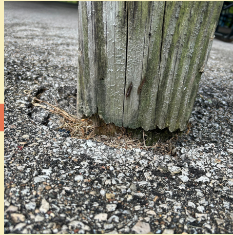
Support Posts Rotting at Base
