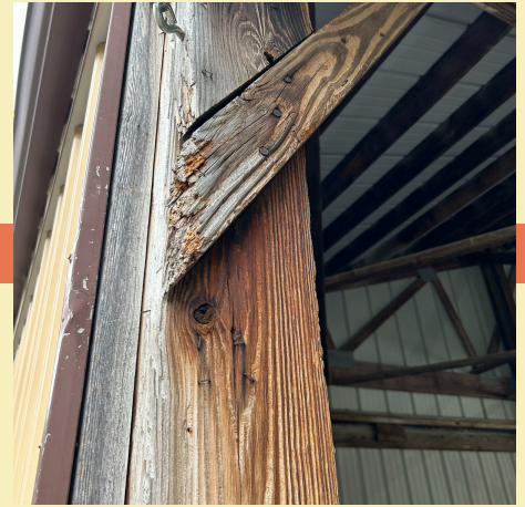
Rotten Support Brackets
