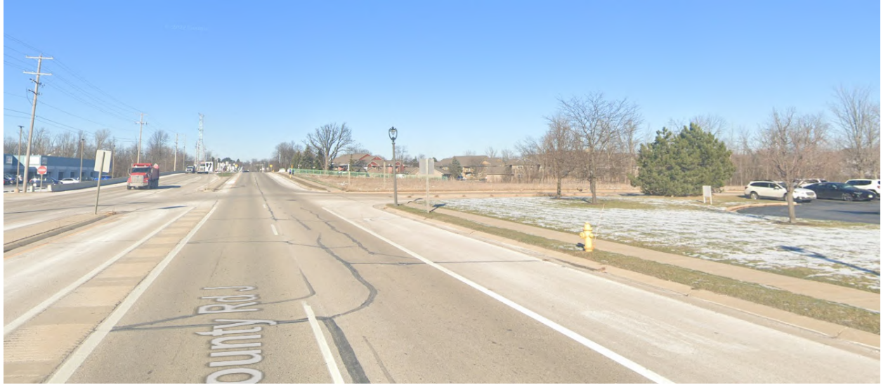
Figure 10: Dedicated right turn lane for NB traffic on WI164
